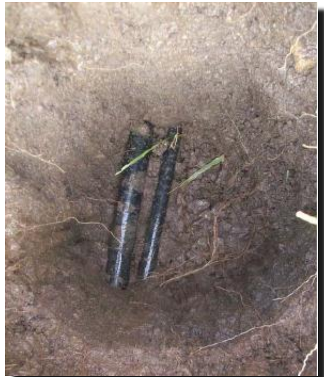
Figure 1 – Exposed Underground Conduit
